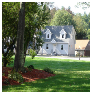
Progress continues on 4 Suburban Road
